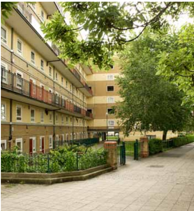
Alpha House, one of several to have been refurbished and reclad
